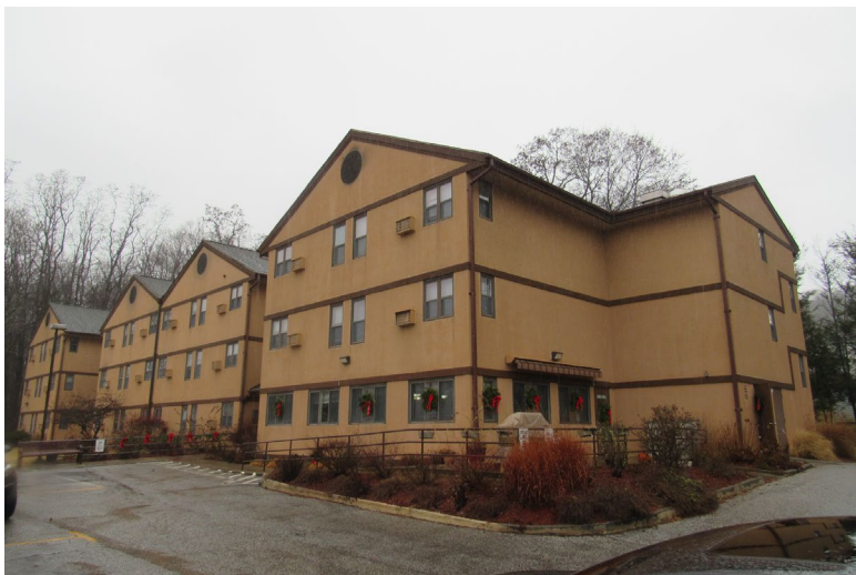
Photo 1: Building architecture as seen at the front elevation
